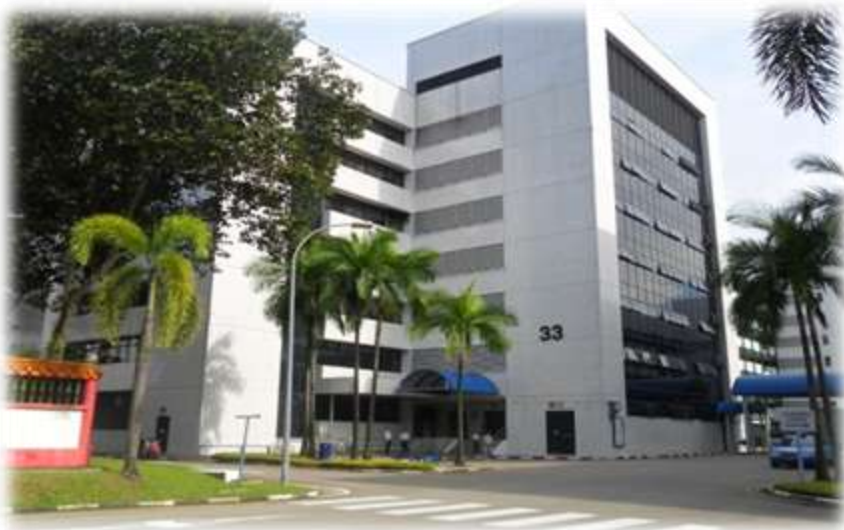
Woodlands Central Cluster before redevelopment
