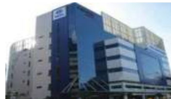
● Tata Communications Exchange
