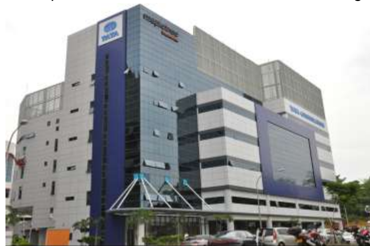
Example of BTS – Tata Communications Exchange
