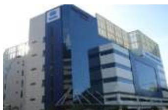
Light Industrial Buildings
